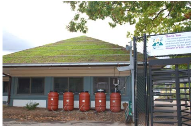
An example of a Green Roof at the Seneca Park Zoo. Photo taken by Laurie Broccolo from the Broccolo Tree and Lawn Care Website at http://www.broccologroup.com/environmental_planning_index.htm
