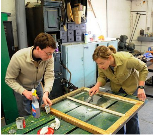
Jayme Breschard re-glazing a historic wood window sash. Photo taken by Jeffrey Chusid, Cornell University's Historic Preservation Planning Program
