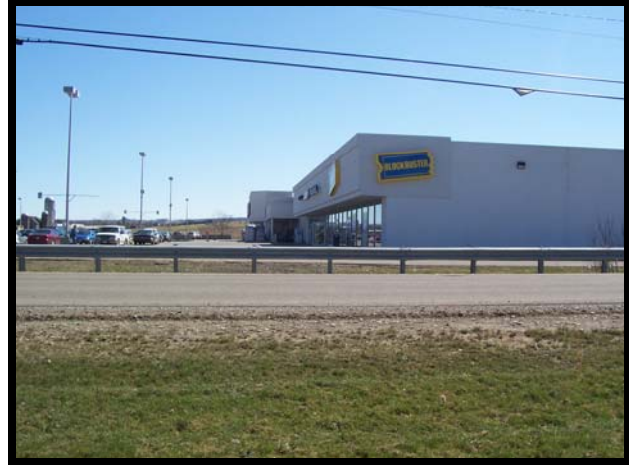
View looking east across Steele Avenue where the proposed new street would intersect with Steele Avenue and the Tops Plaza parking lot.
